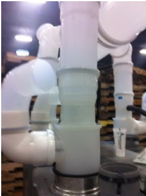
The Valve Installed
